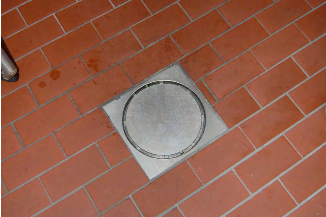
Dairy Plant Floor Drain (First Floor)
